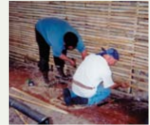
Restoring the plaster walls.
