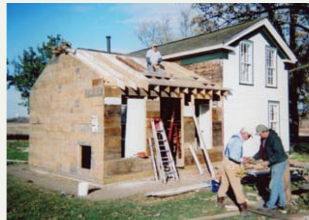
Rebuilding the summer kitchen
