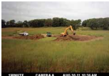
Excavation of sediment from the basin.
