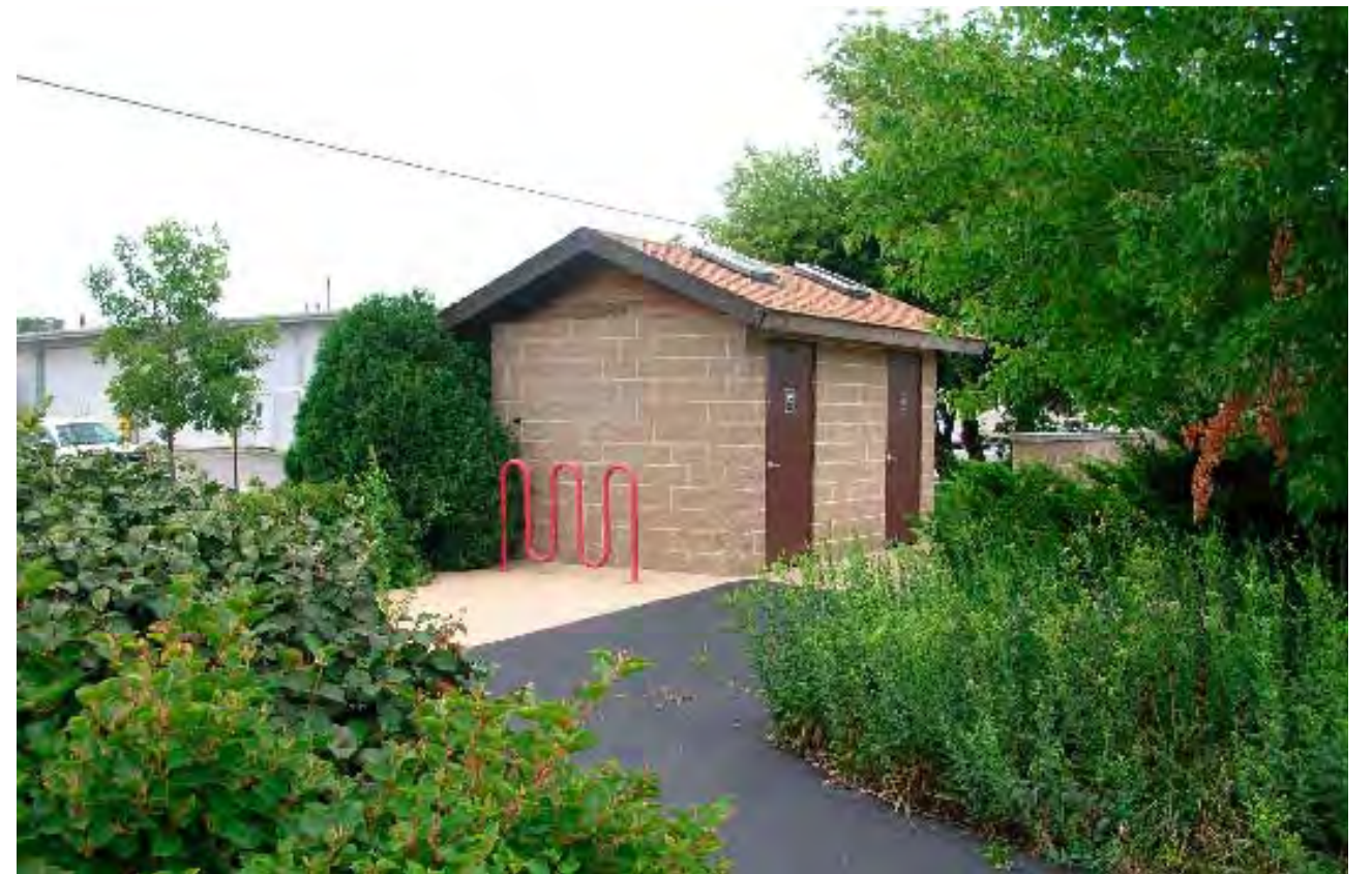
ADA accessible restrooms for trail users
