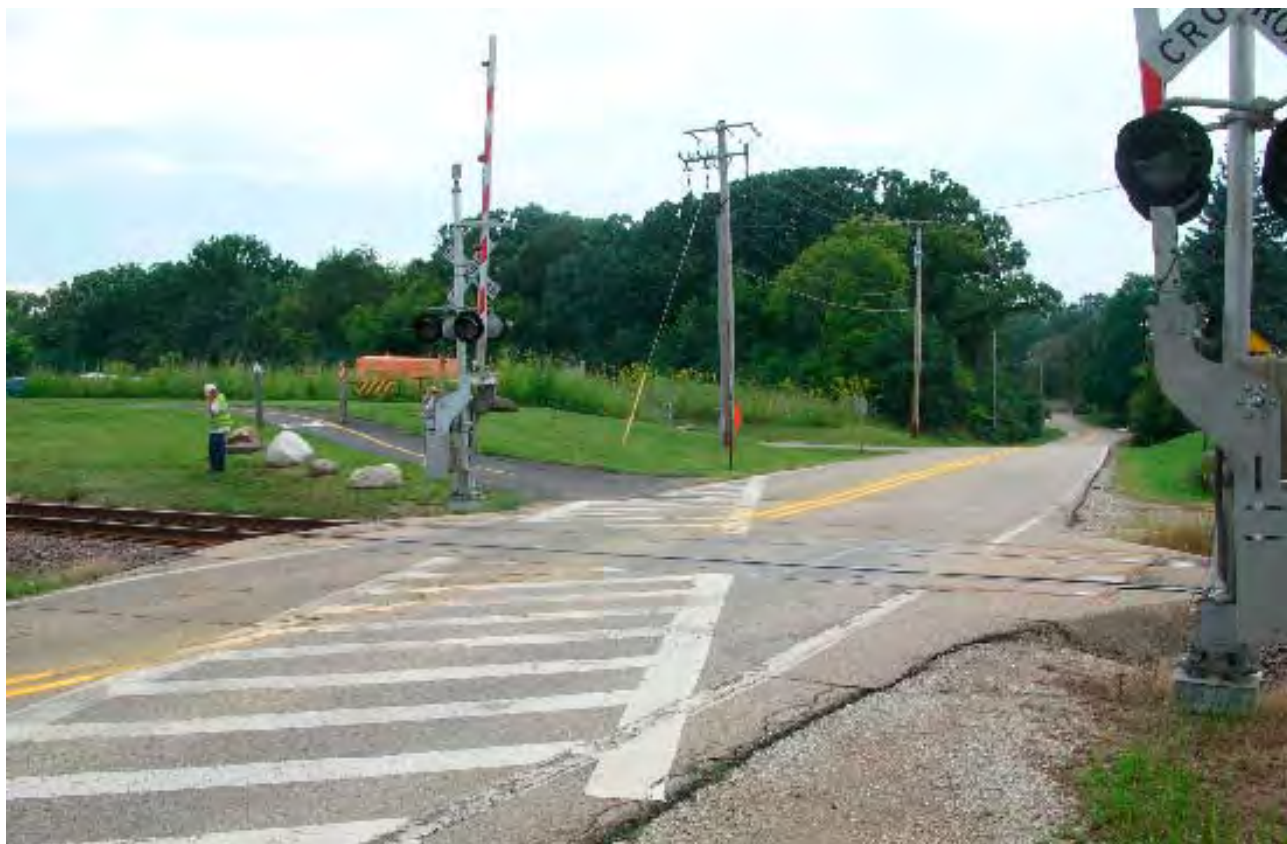
Prairie Trail railroad crossing at Hillside
