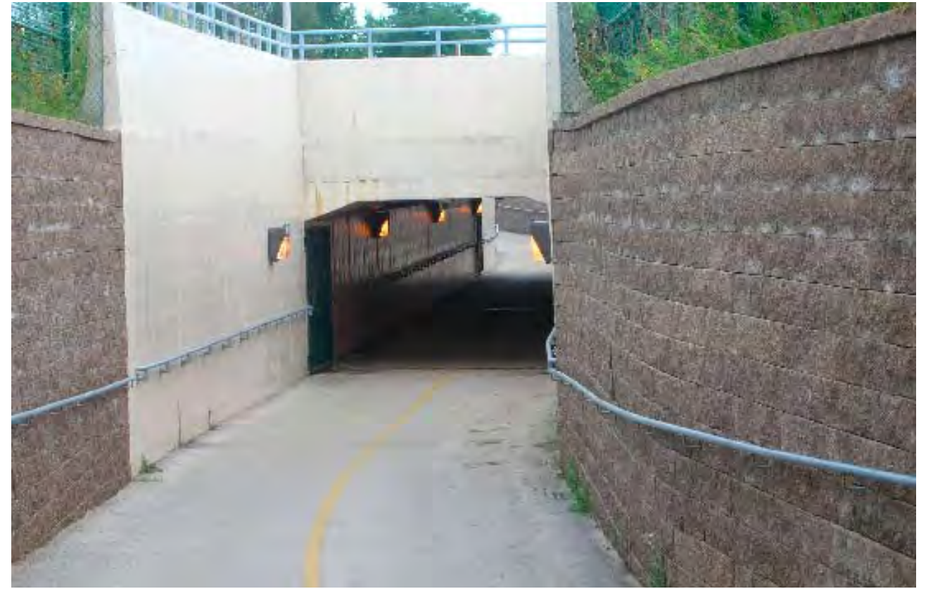
Prairie Trail bridge crossing
